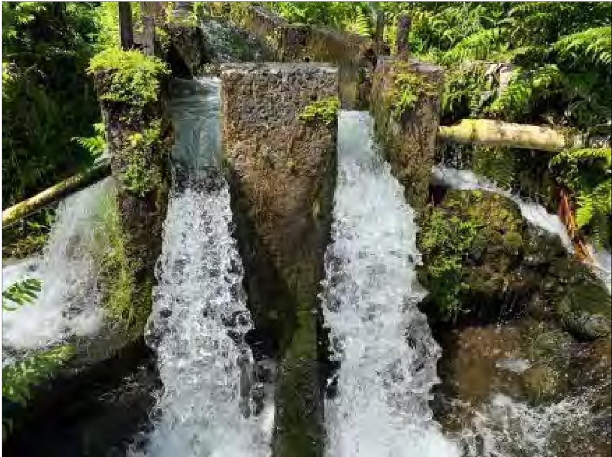
Recommended design solution is to replicate the front facing divider along the right side of the diversion box.
