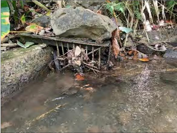
**Debris-clogged drains and 'auwai are typical along this irrigation route.**
