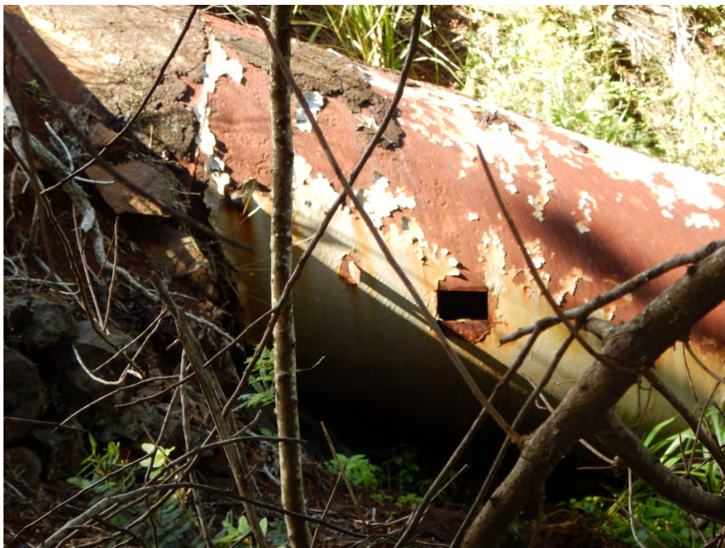
Exhibit 20. O'ahu Ditch - Damaged siphon
