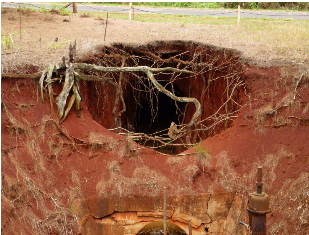
Exhibit 23. O'ahu Ditch - Ditch collapse
