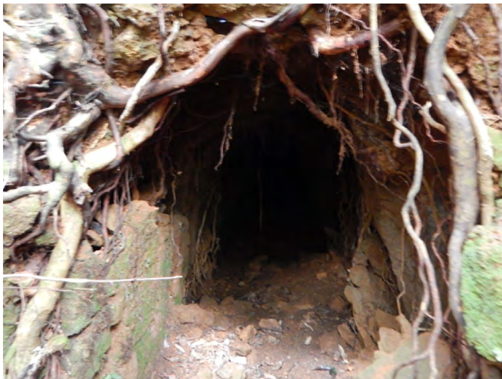
Exhibit 14. Lower Anahola Ditch – Tunnel with root intrusion
