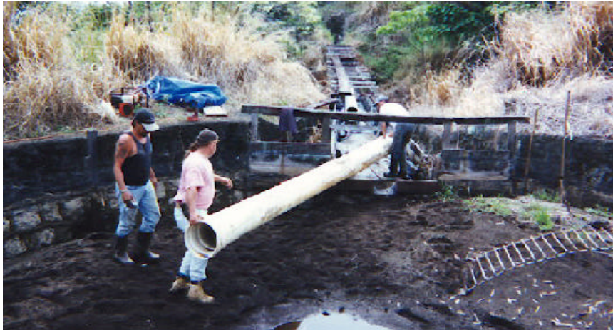
Emergency repair work on the Oshiro Flume, part of the Lower Hamakua Irrigation Ditch on the Big Island. Workers install a 12-inch pipe to replace the old wooden flume, which has deteriorated over the years.
