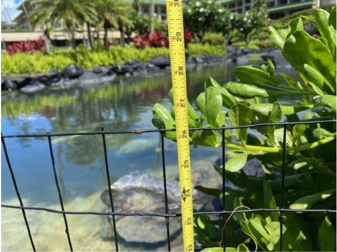
Photograph 14: Depicts Craney Crane's exhibit perimeter fence at two (2) inches by three (3) inches spacing by twenty six (26) inches tall.
