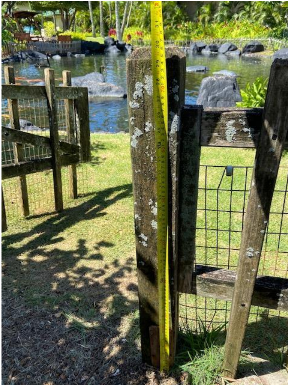
Photograph 1: Depicts Hoku & Mahina's perimeter fence. Thirty (30) inch tall with four (4) to six (6) inch spacing in between wood.
